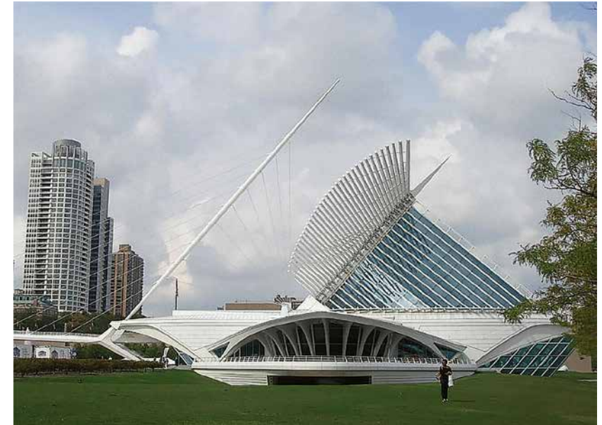
Figure 22: Santiago Calatrava Valls: Milwaukee Art Museum, Quadracci Pavilion, 2001, Wisconsin, USA. (Photo: Andrea Kárpáti)
